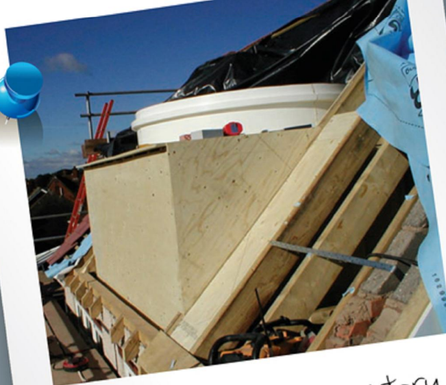
Installation of observatory base
