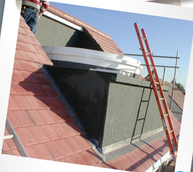
Weather proofing the base
