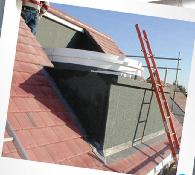
Weather proofing the base
